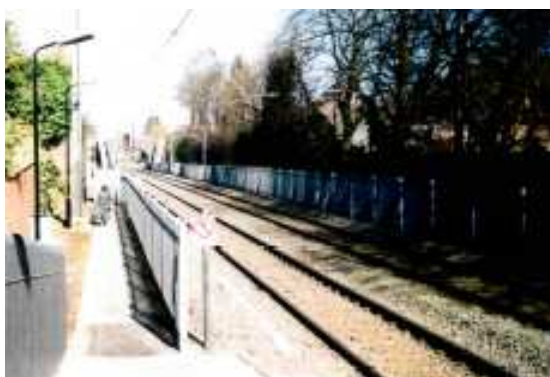
Twin access footpaths at Wylde Green station Sutton Coldfield alongside the 25kV electrified railway.
